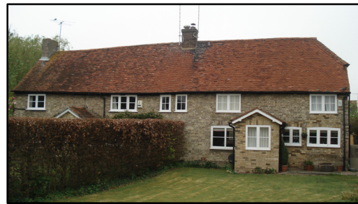
Figure 2. The "Good Intent" Building
