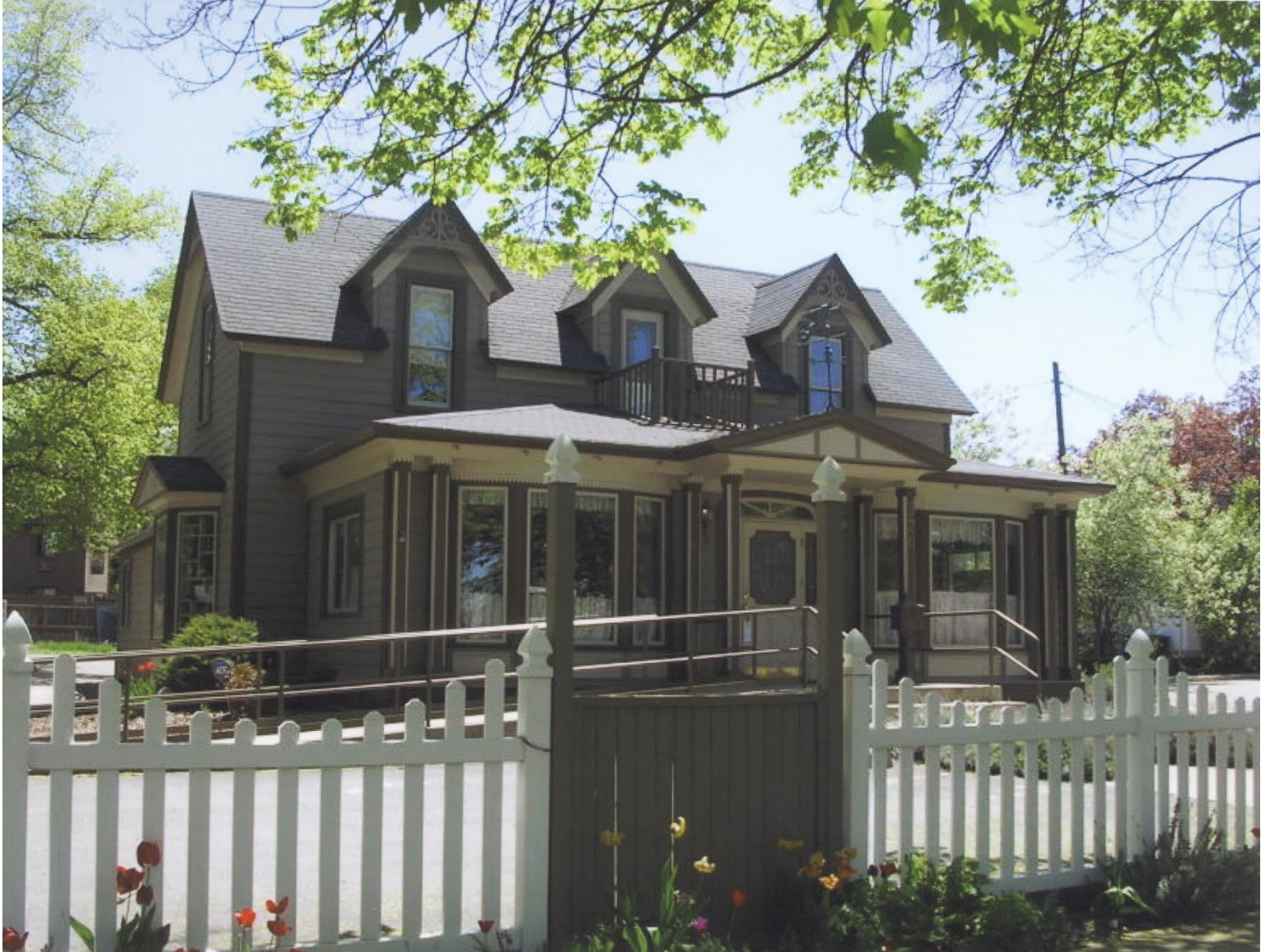
Final Home at 326 North 1 st East, Logan
